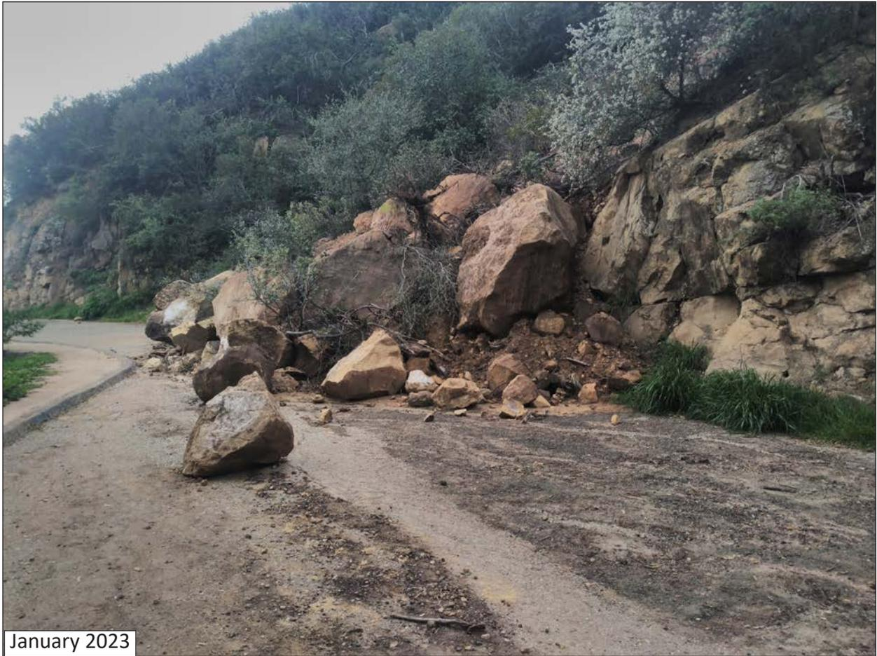
Photograph 5. Spyglass Ridge Road Area 2 with slope failure, looking south.
