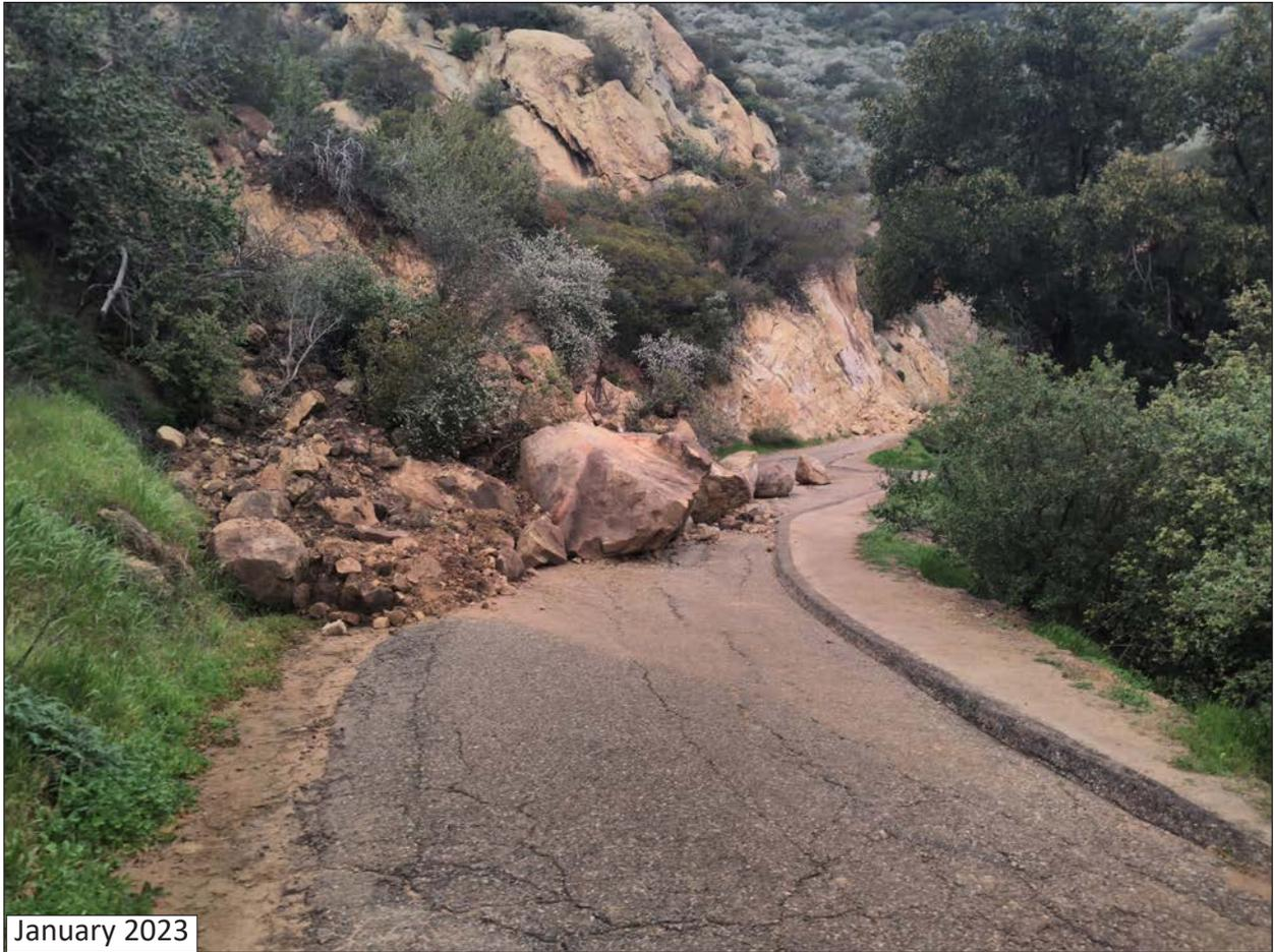
Photograph 3. Spyglass Ridge Road Area 1 with slope failure, looking north.
