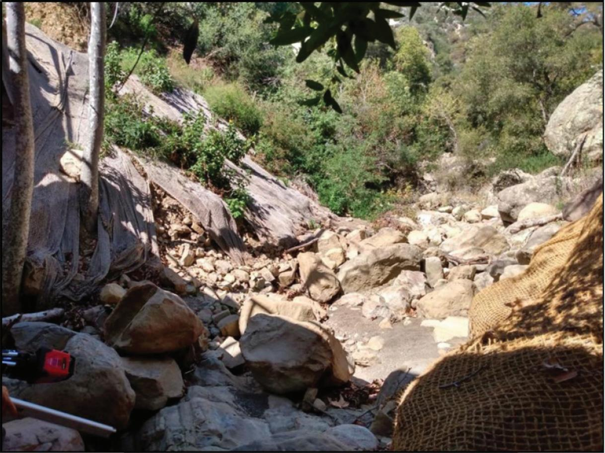
Figure 4: Looking upstream at Creek Site 1 from under the bridge. Sidecast can be seen under netting on both sides of the creek and within the creek bed mixed in with existing rock.
