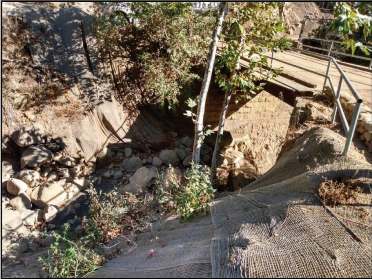
Figure 3: Looking down on Creek Site 1 where sidecast material under netting from top of right bank just upstream of Spyglass Road Bridge.
