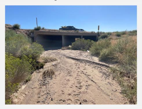
**Photo 6.** View of box culvert along the southeastern portion of the project site, which conveys flows underneath Mojave Drive along NWW- 03. Facing northeast.
