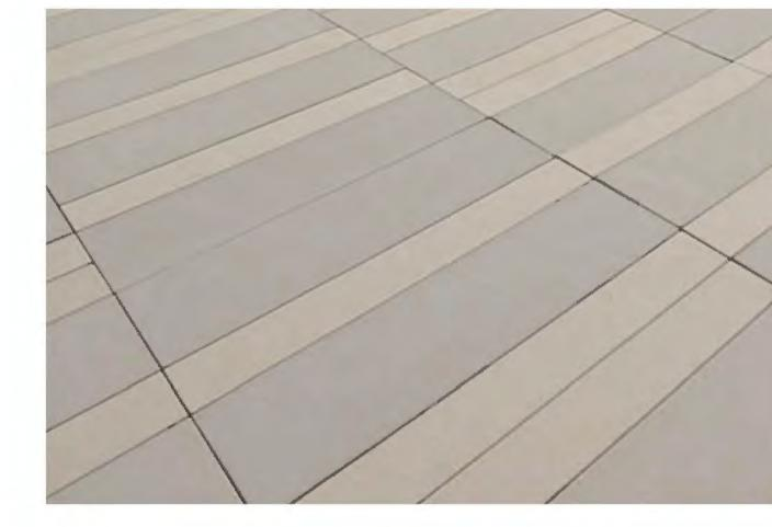
CONCRETE PAVER - TYPE 2 MATERIAL: PRECAST CONCRETE, MORTAR SET SIZE: WIDTHS 6"/12"/24", LENGTHS 48"/60" COLOR/FINISH: LIGHT BUFF/TAN, SANDBLAST
