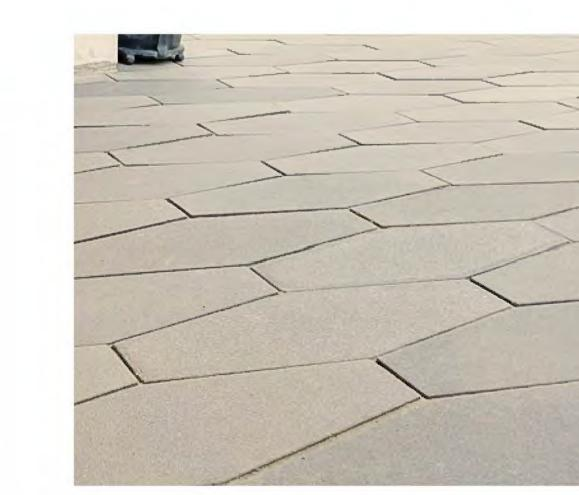
**CONCRETE PAVER - TYPE 1** MATERIAL: PRECAST CONCRETE, MORTAR SET SIZE: 24" X 6" X 12" (DIAMOND) COLOR/FINISH: LIGHT BUFF/TAN, SANDBLAST
