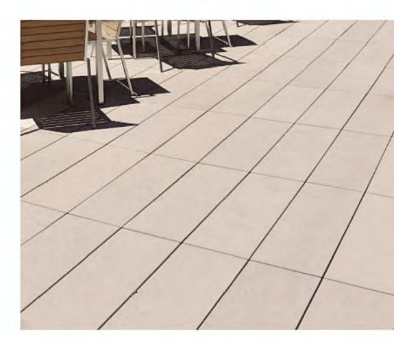
CONCRETE PAVER - TYPE 5 MATERIAL: PRECAST CONCRETE, PEDESTAL SET SIZE: 18" X 48" COLOR/FINISH: LIGHT BUFF/TAN, SANDBLAST
