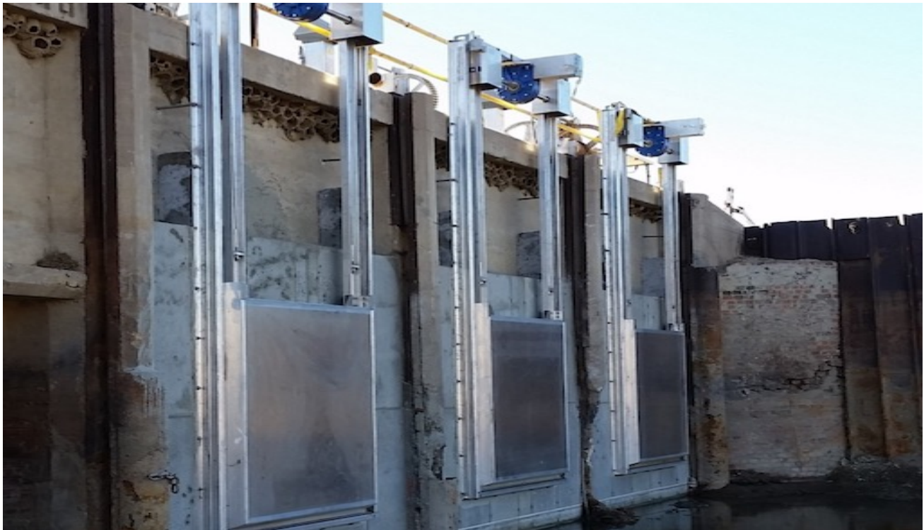
Figure 2-4 Typical Modernized Slip Gates and Check Structure
