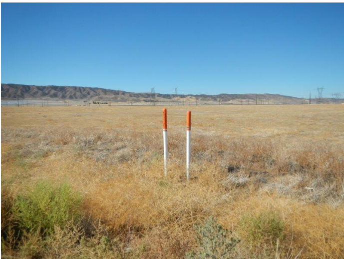
6. View of markers for buried fiber optic lines along eastern property boundary
