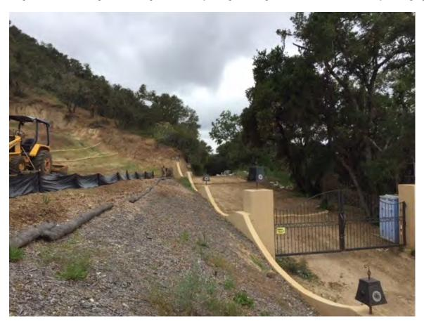
Figure 2. Slope stabilization and sedimentation control measures have been installed and maintained.
