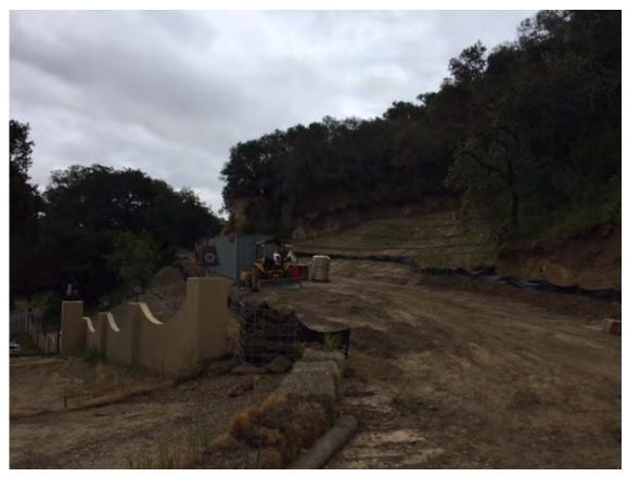
Figure 3. Another view of area near entrance that has been disturbed and exposed by grading activities. Erosion & sedimentation control measures have been installed and maintained.
