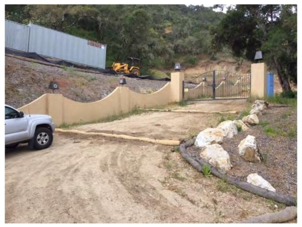
Figure 1. Gated entrance to property off of San Juan Canyon Road. Temporary erosion & sedimentation control measures have been installed to prevent sediment deposition onto public roadway. The plan is to pave the entrance and driveway to the property.
