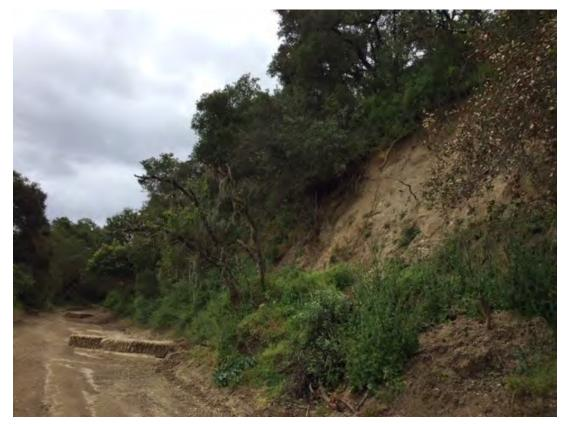
Figure 7. Some tree removal and erosion problems have occurred on disturbed cut slope along property road that was widened. Straw bale sediment traps have been installed along inside edge of road where storm water runoff is occurring.
