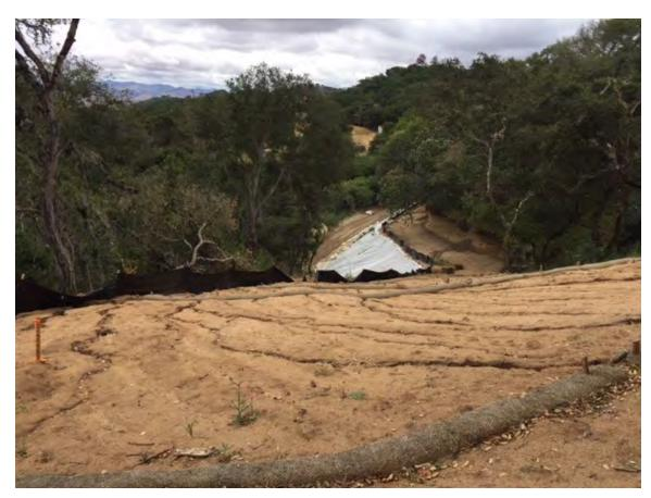
Figure 8. Erosion is occurring on steep upper section of road near the existing homesite. Refer to SWPPP that is being prepared to address erosion and sedimentation control issues.
