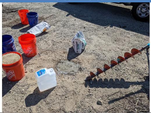
**PHOTO 7:** View of patched boring after sampling completion.
