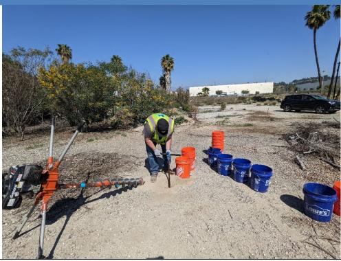
**PHOTO 3:** Hand augering being performed at Boring B-03.
