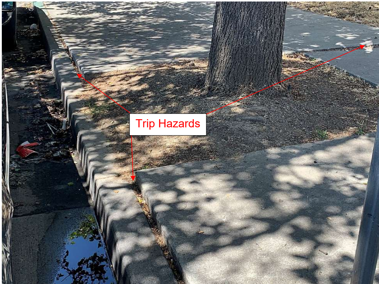
Image #6 – Tree T16, ornamental pear. The lifted sidewalk is creating significant trip hazards in three locations.
