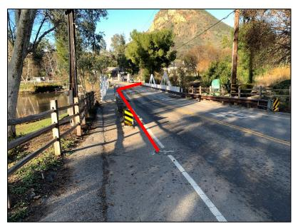
c. Proposed sewer bypass pipe alignment on bridge and shoulder
