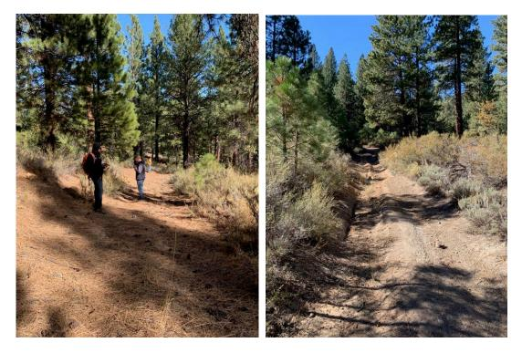
**Photos 2 and 3**. Intersection of cross-country pipeline alignment (left) and existing dirt road (right) where pipeline will be embedded into the road grade under Alternative A or continue downslope directly to the Hirschdale tank and treatment facility under Alternative B.
