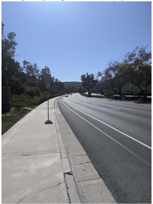
Figure 7-1 shows the existing line of sight looking south on Crown Valley Parkway at the location of proposed driveway. Exhibit 7-1 shows the required sight distance and limited use area and Exhibit 7-2 shows a computer 3-D rendering of the sight distance looking south onto Crown Valley Parkway.
