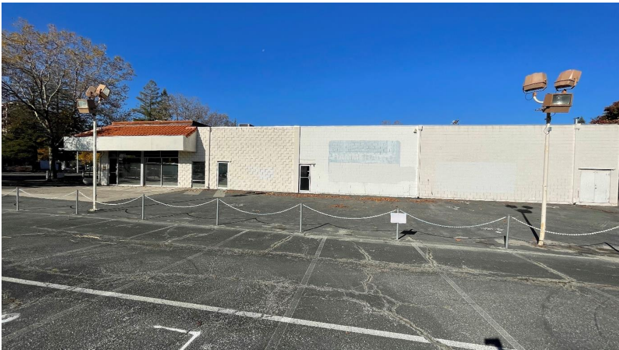
Photograph 6. View of cracked asphalt in the parking lot of the Project Site, facing west. Concrete patches are visible adjacent to the 3017 El Camino Real building.
