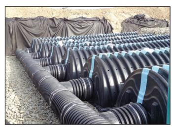
Trimming may only be performed on fully closed end walls (indicated by Number 1 in Fig. 1) or side portal areas (See green circles in Fig. 1 for side portal locations). Pipe may not be inserted into the sidewall of the chamber unless it is within the side portal trim lines. See page 11-12 for more information on trimming side portals.
