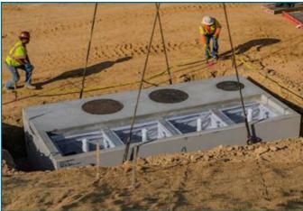
The Modular Wetlands<sup>®</sup> System Linear is simple, easy to install, and has a space-efficient design that offers lower excavation and installation costs compared to traditional tree-box type systems. The structure of the system resembles precast catch basin or utility vaults and is installed in a similar fashion.
