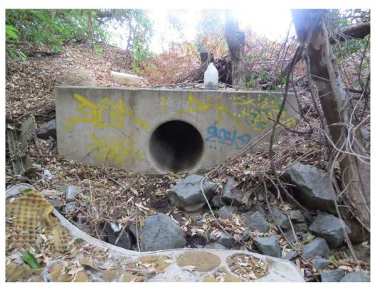
Photograph 12: One of the culverts that conveys flows into Drainage 1 on the southeast corner of the site.
