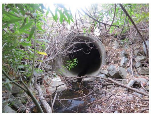
Photograph 11: Main culvert that conveys flows into Drainage 1 on the southeast corner of the site.
