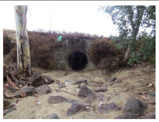
Photograph 17: Looking at the culvert at the western end of Drainage 1 that receives water flows from Drainage 1 and conveys under Murrieta Hot Springs Road.
