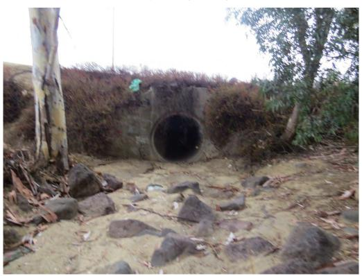
Photograph 26: Looking at the culvert at the western end of Drainage 1 that receives water flows from Drainage 1 and conveys under Murrieta Hot Springs Road.
