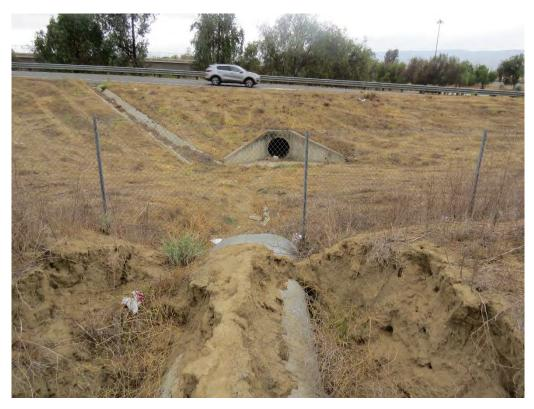
**Photograph 9:** Looking at the culvert that receives water flows from Drainage 2 and conveys water under Interstate 15.
