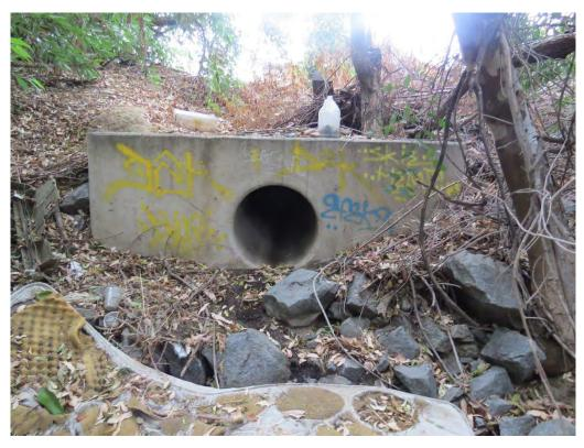
Photograph 21: One of the culverts that conveys flows into Drainage 1 on the southeast corner of the site.
