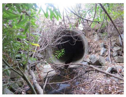
Photograph 19: Main culvert that conveys flows into Drainage 1 on the southeast corner of the site.
