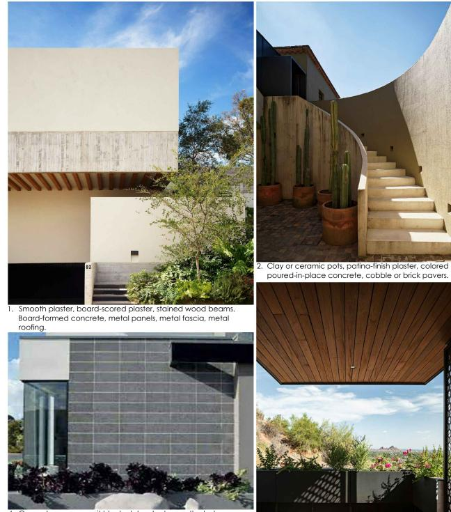
4. Concrete masonry unit blocks, tube steel, smooth plaster.
