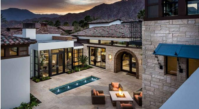
2. Smooth plaster, Stone veneer, Clay tile roofing, steel or iron rails, Canvas awnings, Stone or tile paving, Landscaping.
