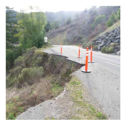
Photo 1 - Adjacent storm damage site at edge of project staging area on Mattole Road
