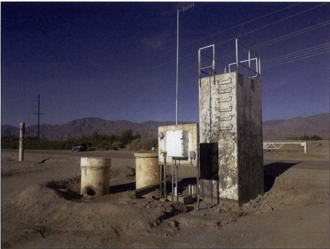
Figure 1. A 14 ft tall box stand, two 36-in diameter standpipes, and meter at 99.8-0.51-6.5 Sta 0+00, intersection of Avenue 64 and Fillmore Street (view to the southwest).
