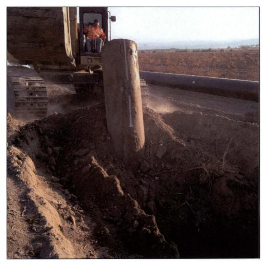
Looking north at removal of existing 27-inch reinforced concrete pipe Irrigation Lateral #99.8-0.51 on Fillmore Street at Station 186+00. Photo taken 8/24/16 by Jim Kreizinger.
