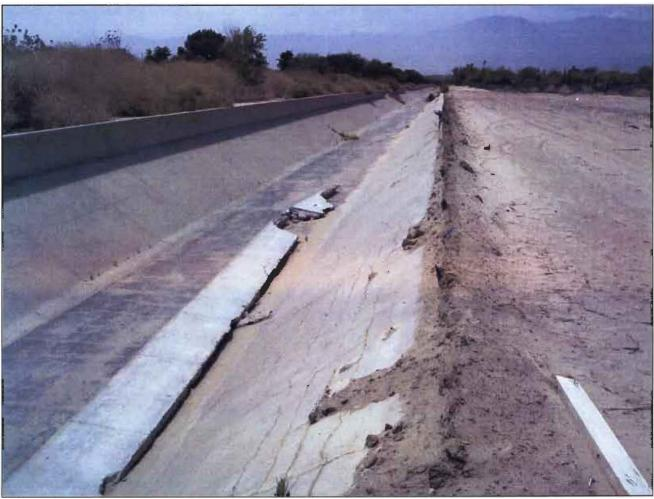
Figure 5. Segment of Wasteway No. 3 on Cabazon Indian Reservation (view to the southwest). Note the collapsed wall laying in the bottom of the wasteway.
