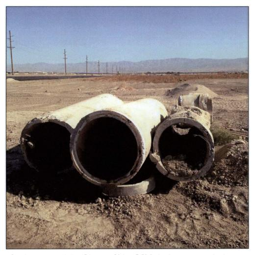
Looking north at existing 27-inch and 30-inch RCP Irrigation removed during both tie-ins for Lateral 99.8-0.51 on Fillmore Street. Photo taken 8/22/16 by Jim Kreizinger.
