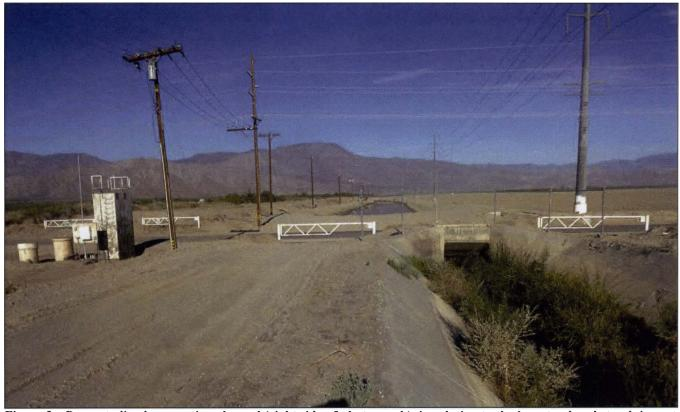
Figure 2. Concrete-lined evacuation channel (right side of photograph), in relation to the box stand and standpipes at 99.8-0.51-6.5 Sta 0+00, intersection of Avenue 64 and Fillmore Street (view to the west).
