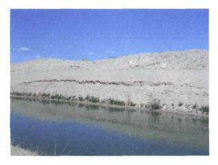
Clay lining eroding from the bank of the canal between Siphon 16 and 17
