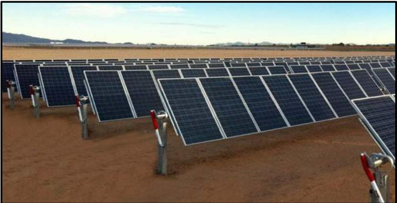
**Figure 5: Example of Photovoltaic Arrays (Single-Axis)**
