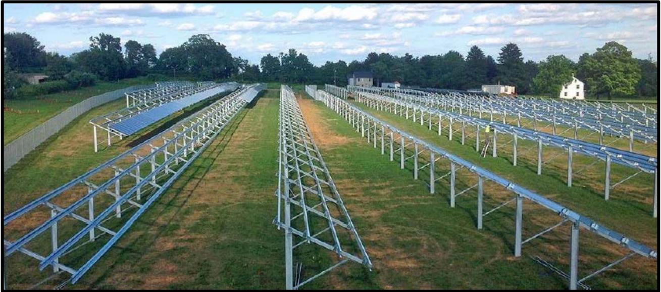
**Figure 4: Example of Photovoltaic Arrays (Fixed-Tilt)**
