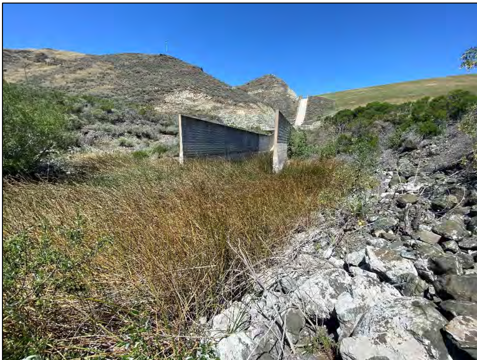
Photo 4. View north/upstream of the rip-rap energy dissipation structure, stilling basin, and instream vegetation (April 12, 2022).
