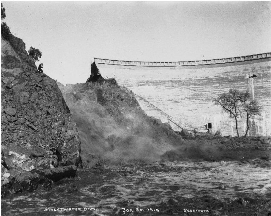
**Figure 10. Water rushing through a break at Sweetwater Dam, Photographer Lee Passmore, 1916, (California Border Region Digitization Project: 1870-1939, San Diego History Center)**
