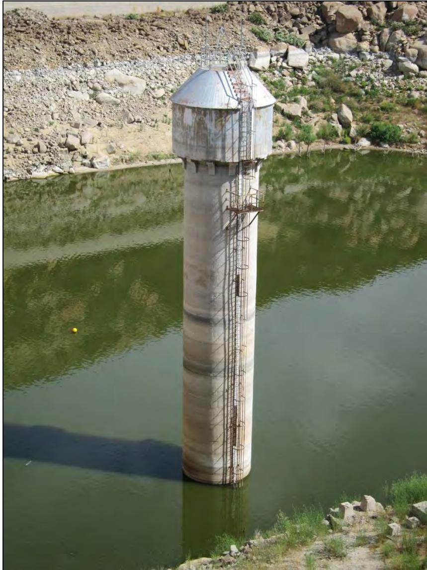
Figure 4. Overview of Morena Outlet Tower; note the concrete footings from the pedestrian footbridge (no longer extant) in the lower right corner (view to northeast)
