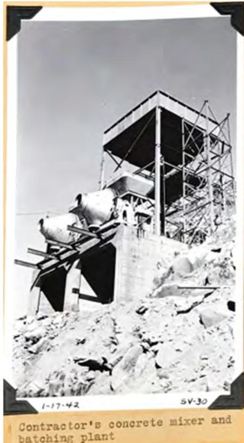
Figure 9. Historical photograph of concrete mixer and batching plant foundation.
