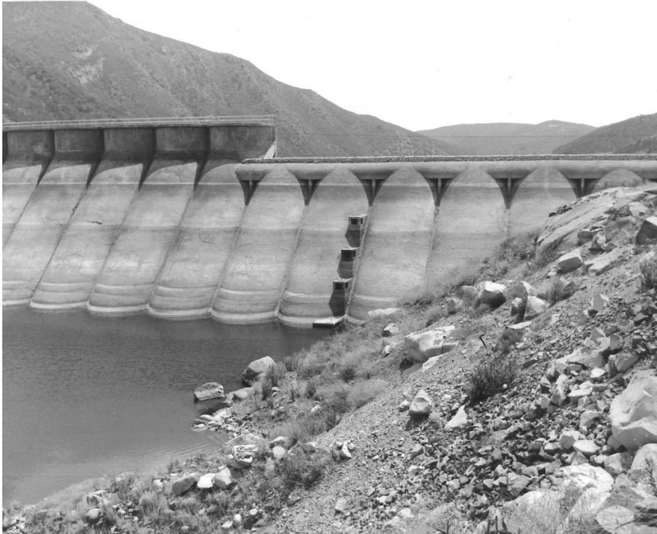
Figure 20. Sutherland Dam, upstream face showing multiple arch type of construction, 1954. (City of San Diego Public Utilities Department Archives, Box 10, Folder 103)
