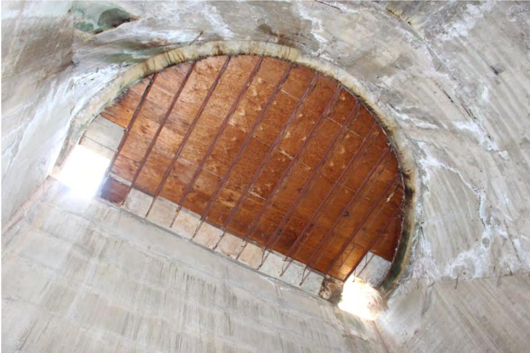
Figure 9. Supporting joists of plywood for the roof structure, view looking upwards, IMG 0522
