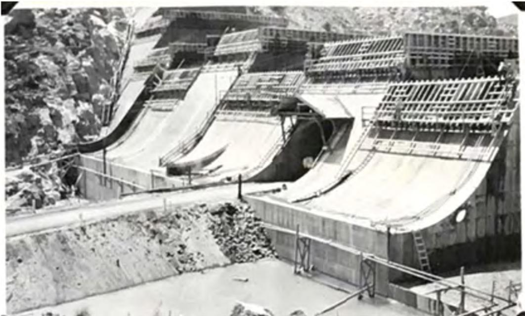
Figure 16. Dam construction showing tunnel through base of the dam, August 1942
