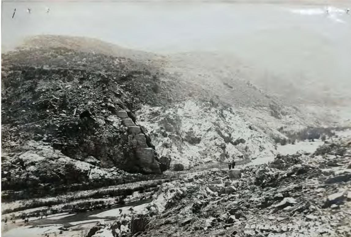
Figure 8. Remains of the Original Dam Following the Collapse in 1916 (City of San Diego 1919)
