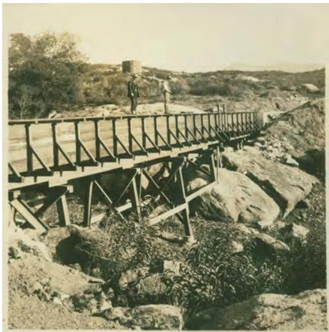
Figure 7. Photograph showing wooden flume construction supported by bridges, near Bee Canyon, 1909 (M.M. O'Shaughnessy Photograph Collection, NUI Galway Digital Collections)
