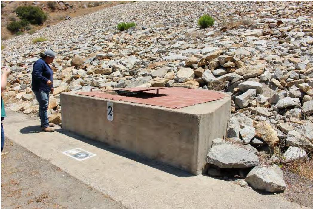
Figure 4. Well access port on downstream access road for dam, looking northeast (IMG 2062)
