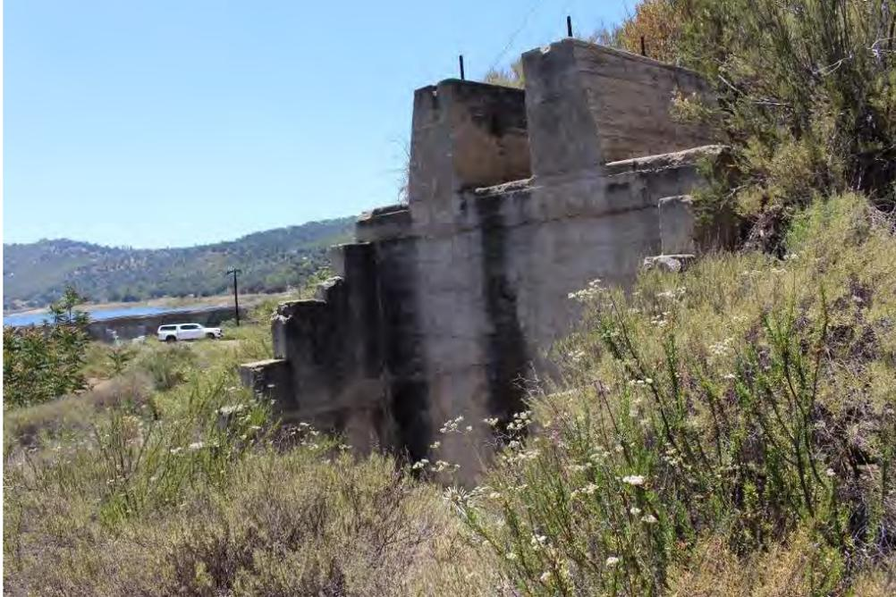
**Figure 11. Stair-stepped footing, looking south with Sutherland Lake in background, IMG\_1434**
