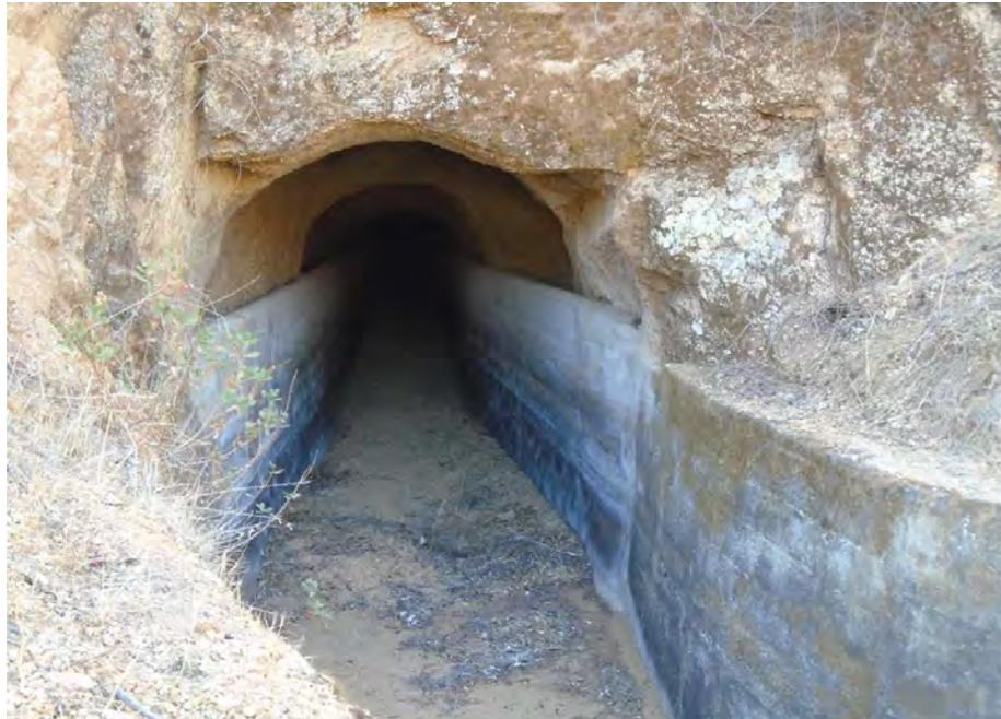
Figure 2. Concrete lined tunnel entrance, DSC00679
