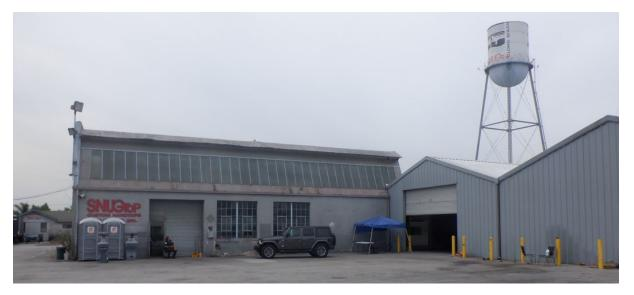
Photo 7. Eastern wing along Harbor Avenue with ribbon skylights and enframed metal sash windows (center). At right are two warehouses added to the northeast corner of the building complex in 2003. (Michael Baker International 9/9/2022)
