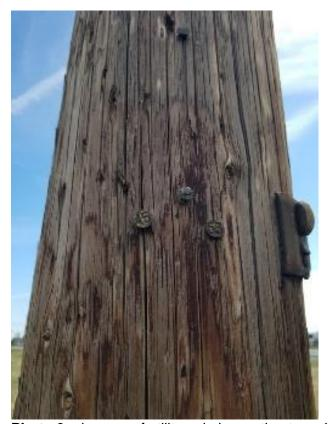
Photo 3: close up of utility pole inspection tags; UTM 11S 458051mE 3777254mN
