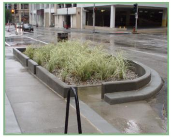
adsorbed, and biodegraded by the soil and plants. Stormwater planters are typically planted with native, drought-tolerant vegetation that does not require fertilization and can withstand wet soils for at least 96 hours.
