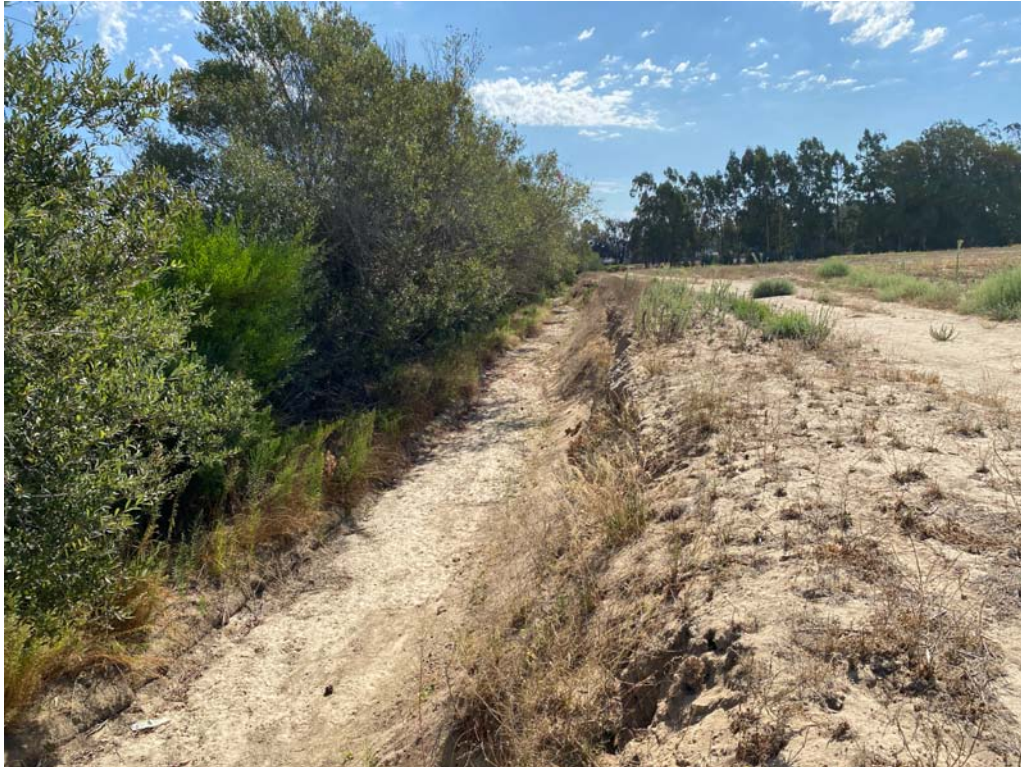
Photo 7. Easterly view of storm drainage ditch showing steep banks and dry channel during the summer months.
