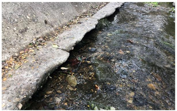
**Photograph 5.** View of the eroded base of the existing slope protection infrastructure, facing southwest (downstream).
