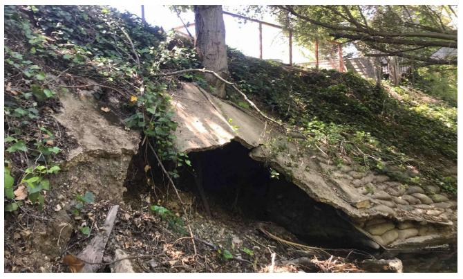
**Photograph 1.** View of the south bank of San Luis Obispo Creek where the concrete infrastructure has been undercut and eroded by water flow (facing south, May 3, 2022).
