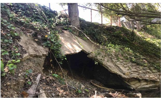
**Photograph 5.** A closer look at the south bank of San Luis Obispo Creek where the concrete infrastructure has been undercut and eroded by water flow (facing south, May 3, 2022).
