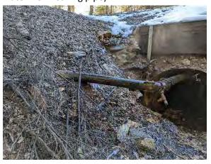
P01 – Broken water pipe in OW08 looking south
