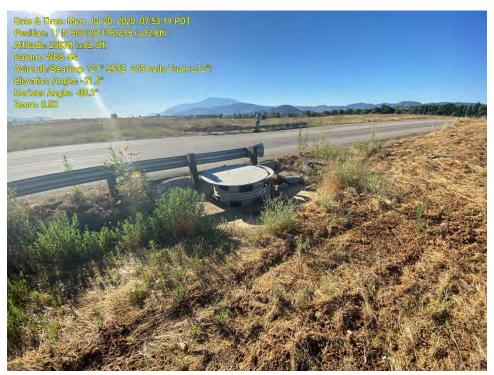
**PHOTOGRAPH 3:** The westside of Pennsylvania Avenue where storm runoff entered a standpipe connected to the culvert where Feature A began.
