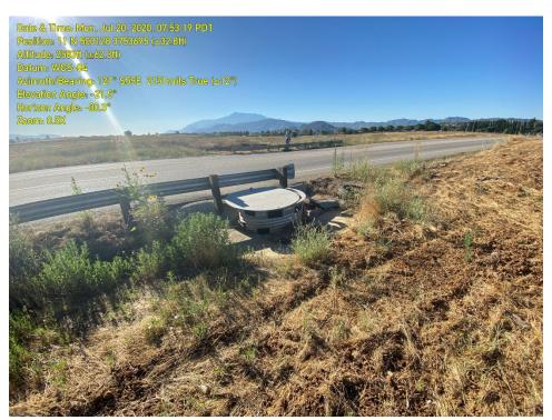
**PHOTOGRAPH 3:** The westside of Pennsylvania Avenue where storm runoff entered a standpipe connected to the culvert where Feature A began.
