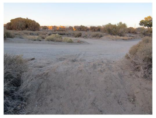
Photograph 14: Ending of the onsite drainage feature where it begins to sheet flow at the dirt access road before flowing across.
