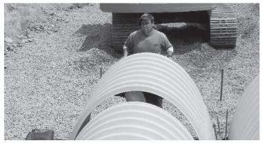
Continue installing chambers by overlapping chamber end corrugations. Chamber joints are labeled "Lower Joint – Overlap Here" and "Build this direction – Upper Joint" Be sure that the chamber placement does not exceed the reach of the construction equipment used to place the stone. Maintain minimum 9" (300 mm) spacing between rows.
