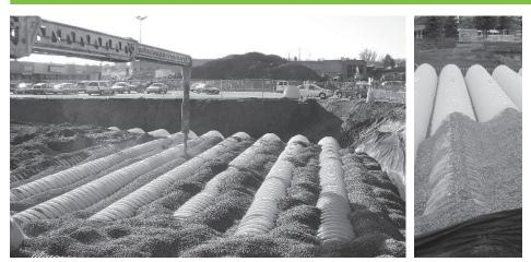
Initial embedment shall be spotted along the centerline of the chamber evenly anchoring the lower portion of the chamber. This is best accomplished with a stone conveyor or excavator reaching along the row.
