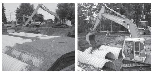
No equipment shall be operated on the bed at this stage of the installation. Excavators must be located off the bed. Dump trucks shall not dump stone directly on to the bed. Dozers or loaders are not allowed on the bed at this time.
