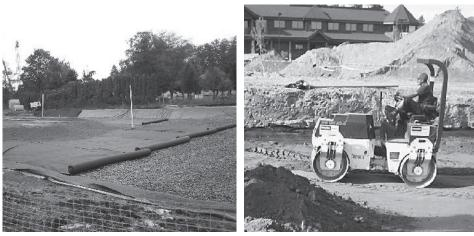
Install non-woven geotextile over stone. Geotextile must overlap 24" (600 mm) in. where edges meet. Compact at 24" (600 mm) of fill. Roller travel parallel with rows.
