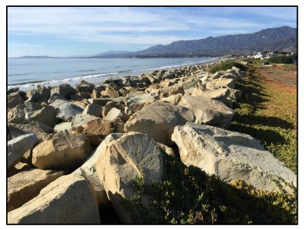
Photo 11. The revetment protects Sand Point Road residences from Pacific Ocean storm surges. View northwest, November 11, 2017.
