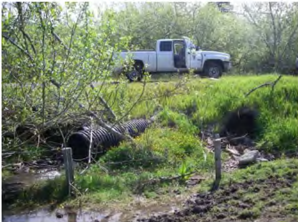
Figure 5. Crossing #4 at Cedar Lodge Lane is a series of four undersized culverts, one of which is overgrown and plugged with debris. This crossing will be replaced with a culvert that meets all fish passage criteria and passes the 100-year flows.
