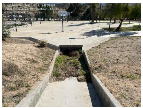
**PHOTOGRAPH 9:** A concrete channel leading down to the culverts of Feature A<sub>2</sub> under the sports complex.
