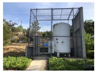
**Photograph 7.** View of the onsite oxygen tank.
