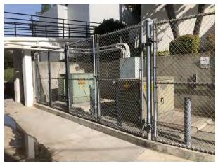
**Photograph 6.** View of the onsite pad mounted transformers.
