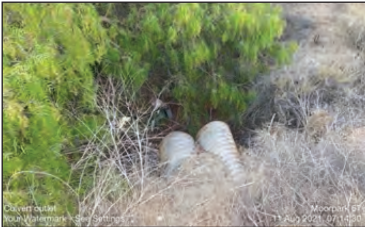
Photo 2C: View looking south at the culvert pipe outlet that allows the water to flow underneath a dirt road.
