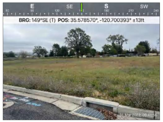
Photo 6. View of storm drain and culvert to direct flow from Nutwood Circle into shallow drainage basin located off-site (north) of the Project Site.
