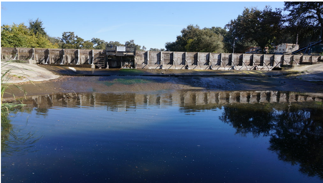
Figure 4. The 8-ft flashboard dam installed on upstream sill of the Bellota Weir.
