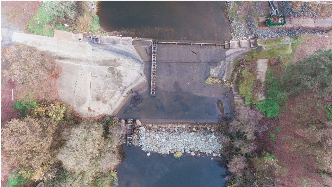
Figure 5. Overhead view of the Bellota Weir with the temporary fish ladders installed.
