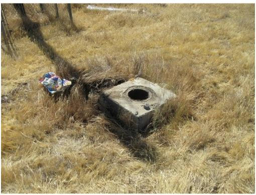
Photo 13: View of a non-operational apparent former agricultural water well located in the northeastern portion of the subject site.
