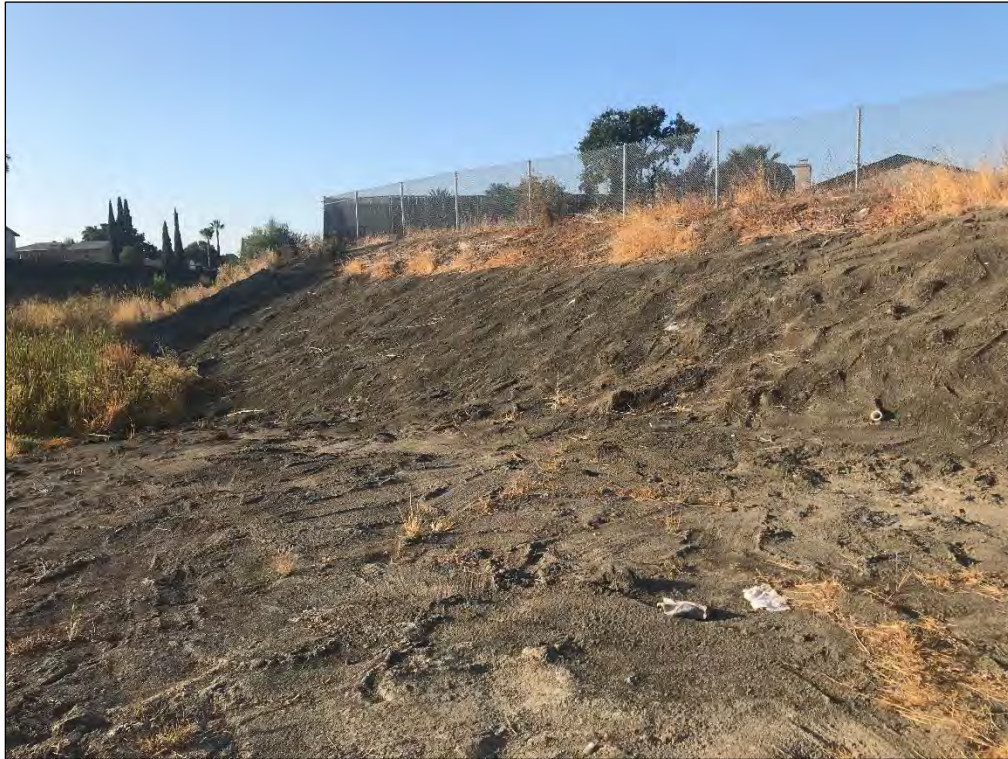
Photo 11. Flood control channel lined with armoring substrate at proposed outfall location (aspect southeast; 8/26/21).
