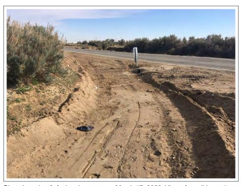
Photo Location 6, facing downstream. March 17, 2022. View of conditions where stream channel flows toward 8th Street along eastern site boundary. Note that road shoulder is graded to allow water to flow off road into channel. Small culvert is evident that allows water to drain eastward under 8th Street.
