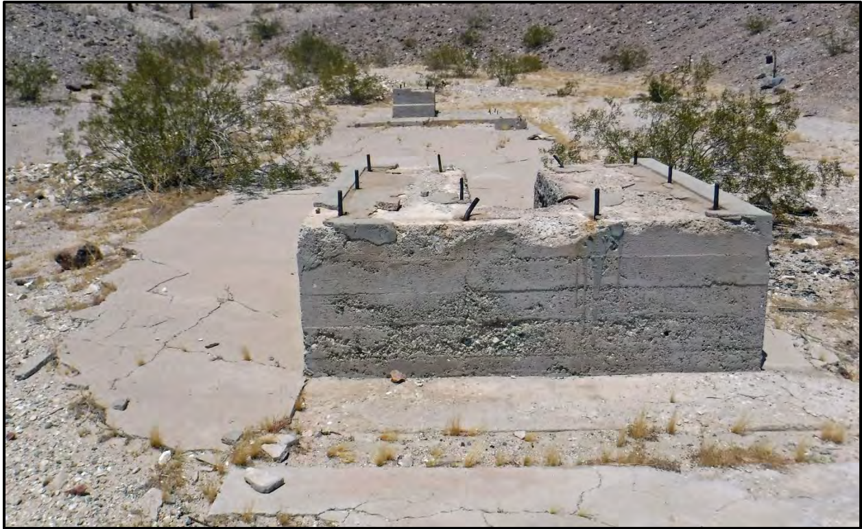
Figure 19. Large Concrete Slab Foundation with Equipment Footings.
