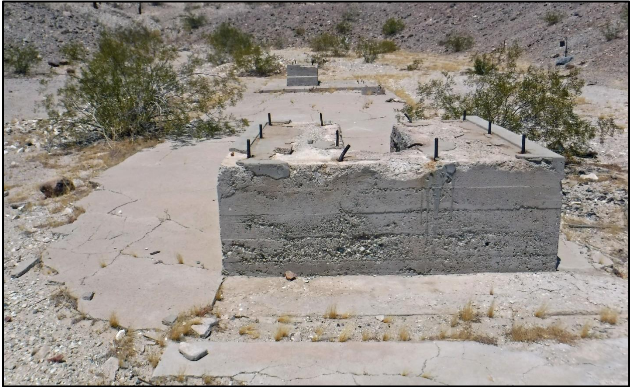
Figure 19. Large Concrete Slab Foundation with Equipment Footings.
