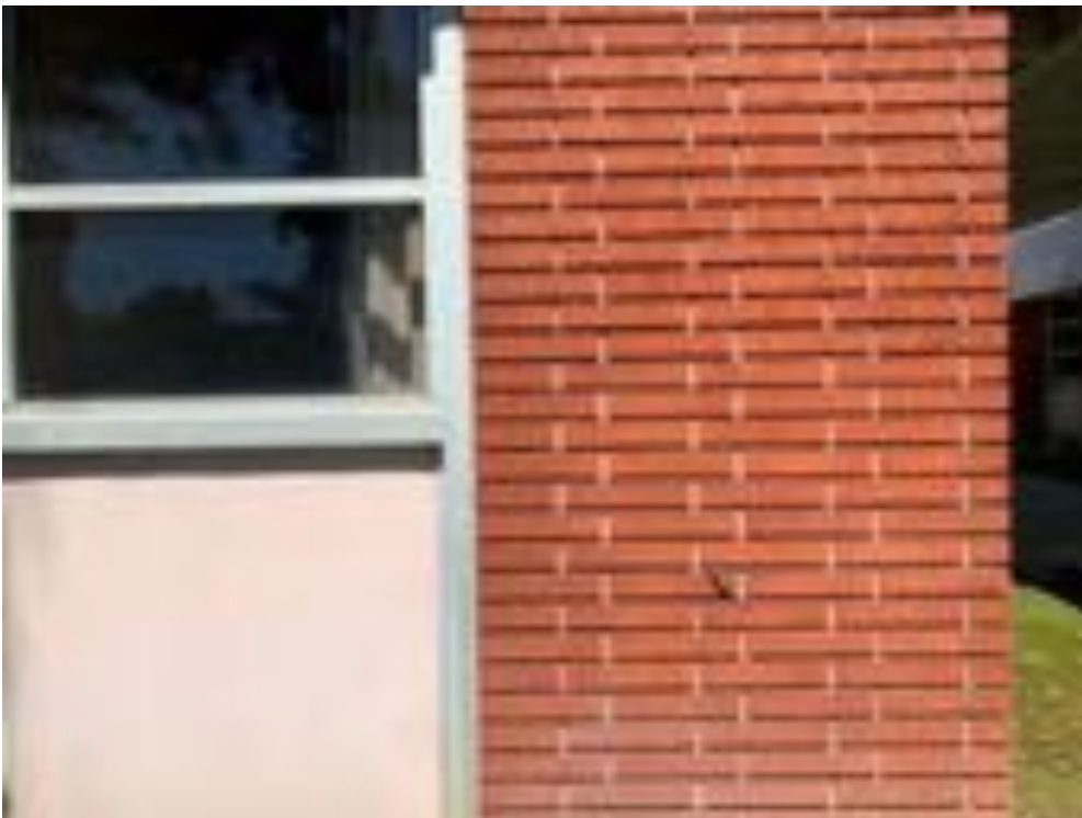
64. Brick stretcher pattern detail
