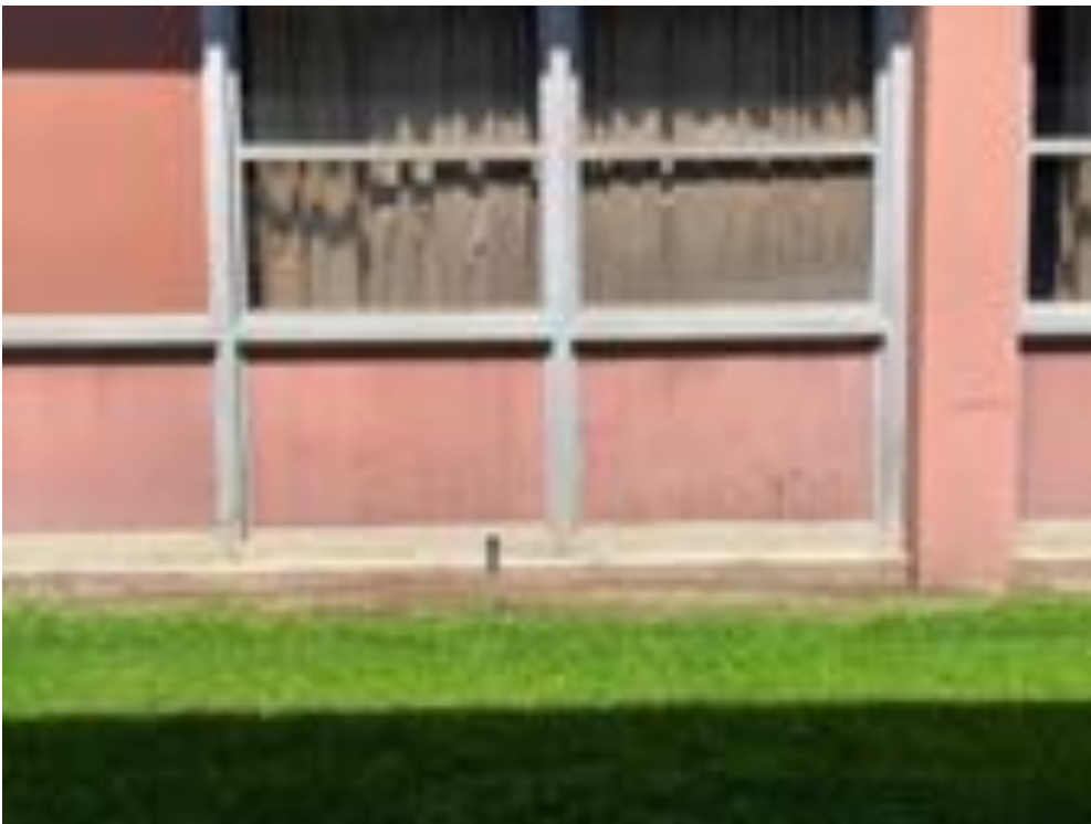
62. Window and concrete panel bulkhead detail
