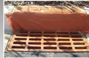
Combination inlet with magnetic rear guard attachment
