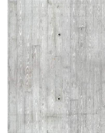
M-01 = VERTICAL BOARD FORMED CONCRETE
