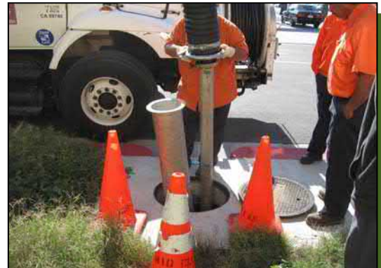
Insertion of vacuum hose into separation chamber.
