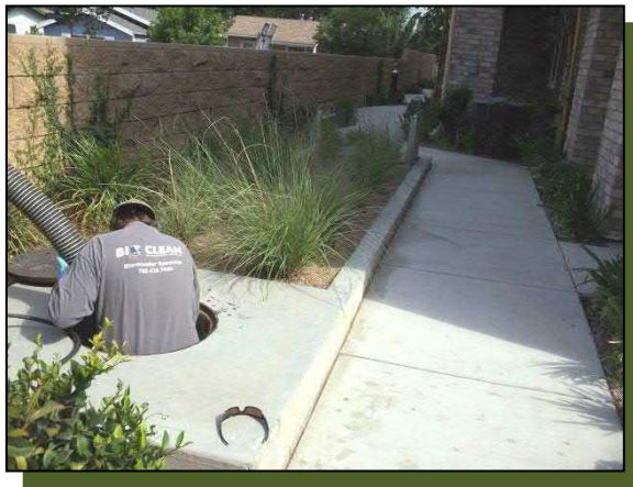
Vacuuming out of media filters.
