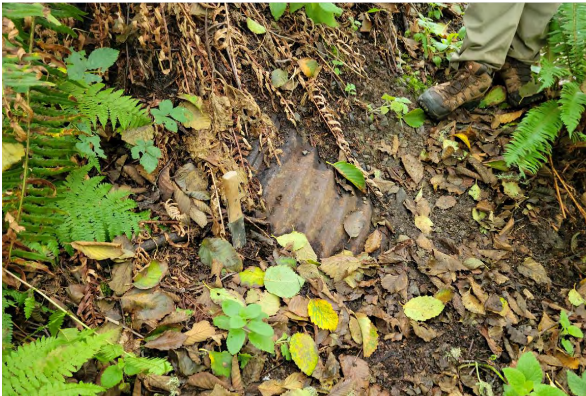
Photograph Location No. 8, Photo A: Corrugated metal culvert that appeared to be related to ephemeral road drainage for Hwy 101.
