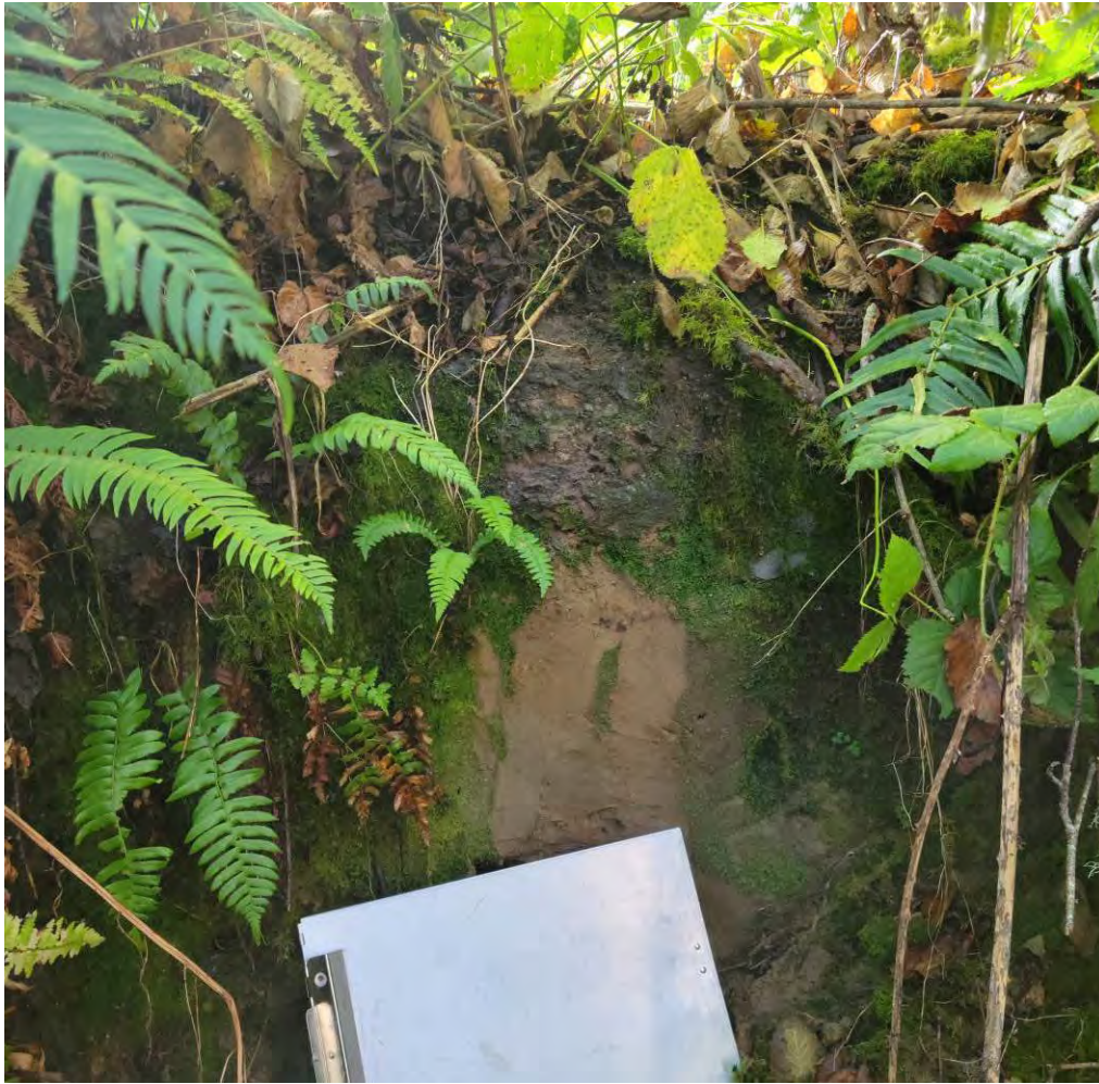
Photograph Location No. 8, Photo B: An exposed section of buried road base resting on sand, immediately downslope of the corrugated metal culvert.
