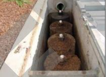
Cartridge Media Filter Source: Contech Stormwater Solution, Inc.
