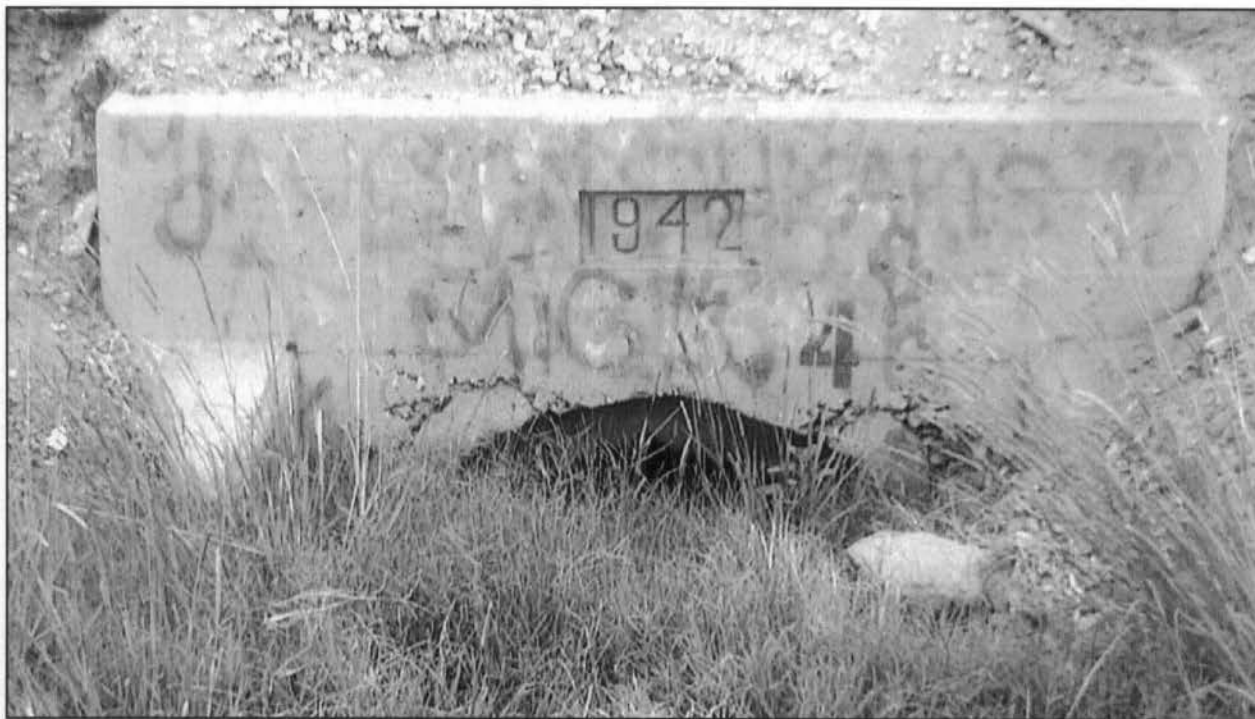
Old concrete culvert across the railroad bed
